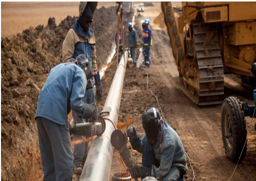
Picture 3 – Engineers installing a brand new pipeline from Enbridge Inc. USA in Angola oil field in Luanda
