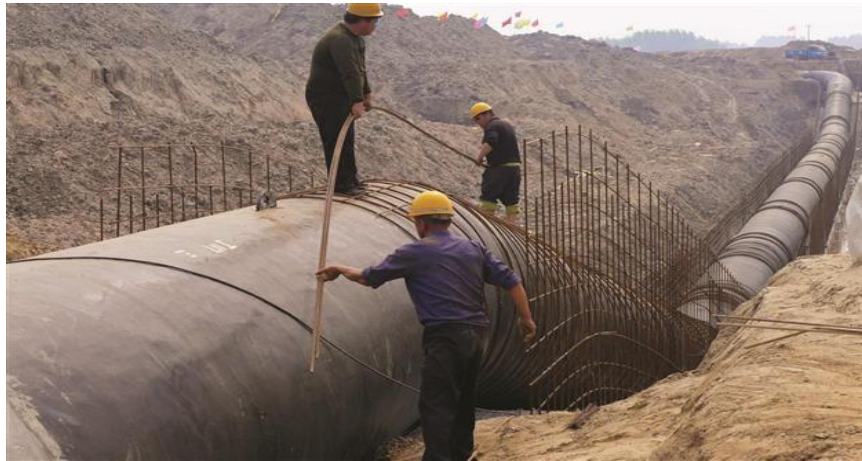
Picture 2 – Engineers positioning the hard coated Enbridge pipelines
