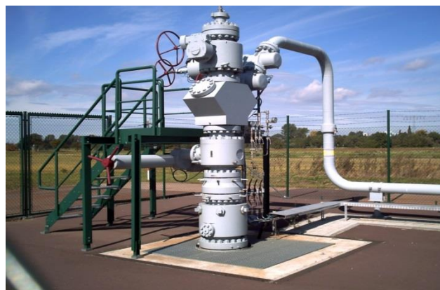
Picture 2 – Newly replaced geothermal wellhead by Paker Company in Yemen's oil field
