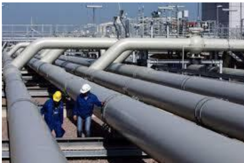
Picture 3 – Newly constructed pipelines with improved coatings to prevent wares and rapturing
