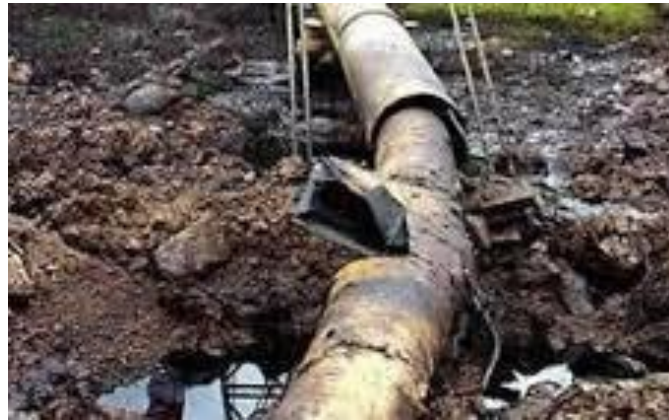
Picture 2 – A ruptured pipeline caused by vandalism leading to large volumes of oil leaks in Nigeria
